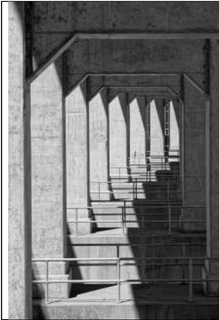
Fort Peck Spillway By Guy Bralley
